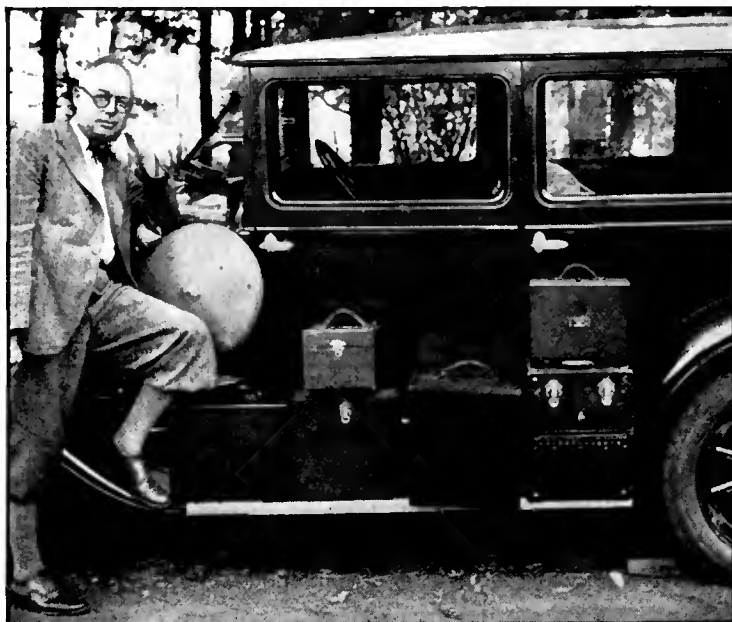
The portable service laboratory of Waldo Todd Pratt, which makes it possible for him to carry on almost any service work under the actual conditions experienced by the set user.
